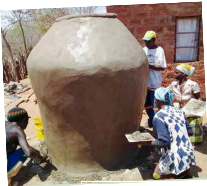
Soft Food Alliance's first rain jar. Local builders Charles Nyoni and Alfred Sibanda plastering the rainwater collection jar along with permaculture trainees.
